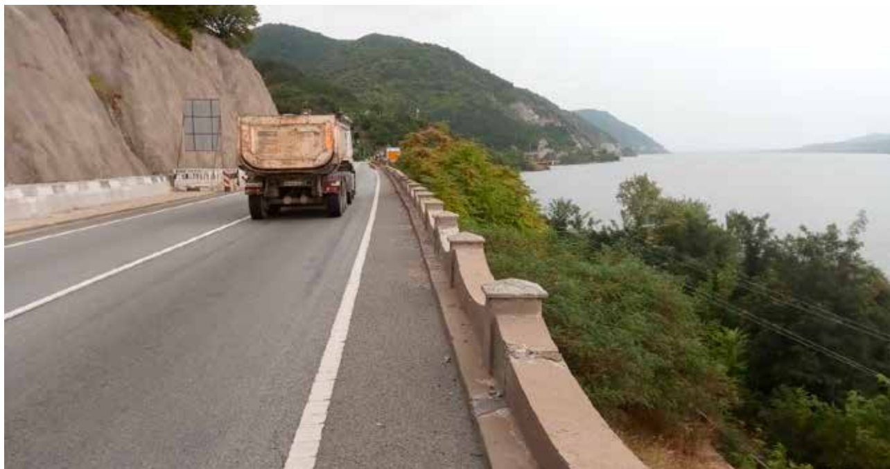
Daily section 66: Orsova - Drobeta-Turnu Severin. To verify whether there is a possibility to construct a cycle path at a lower level, next to the railroad track. Otherwise, an extension that overhangs partially could be constructed at the carriageway level.
