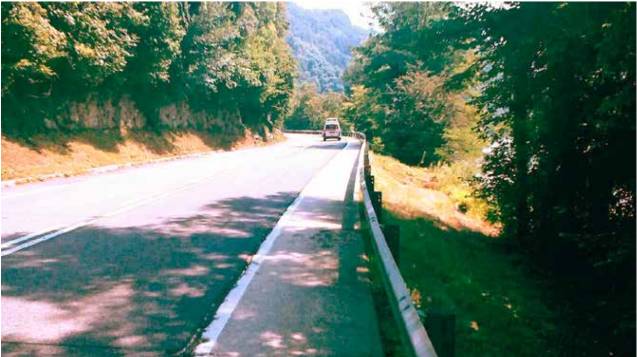
Paved shoulder on road number 3 between Grein and Hirschenau (daily section 17) – too narrow for safe cycling outside built-up area, effective width further reduced by safety barrier.
