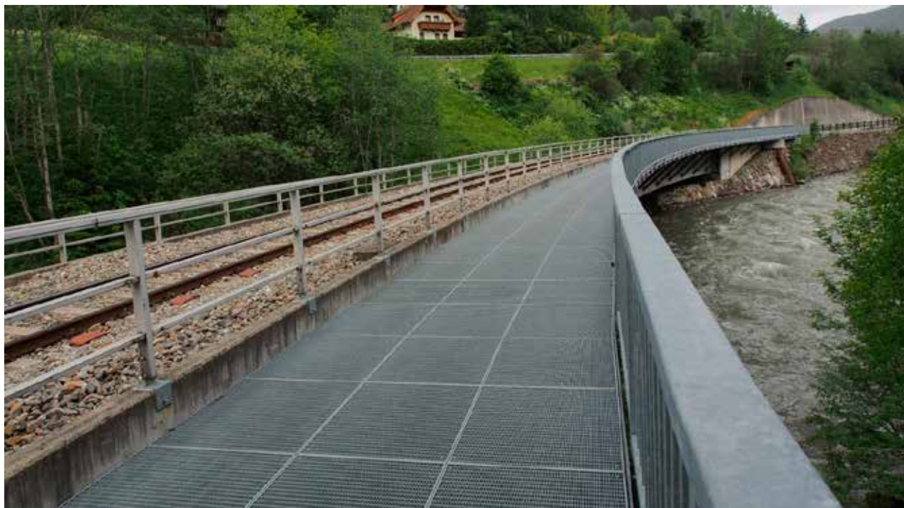
Cycle path attached to railroad embankment – one of the possible solutions for daily section 66. Photo from Murradweg between Tamsweg and Madling (Austria).
