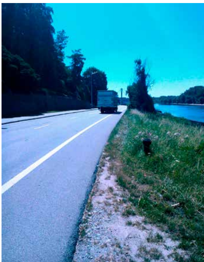
Very high traffic on public road close to Deggenu (section 11). Painted cycle lane/paved shoulder with width of less than 1.5 m.
