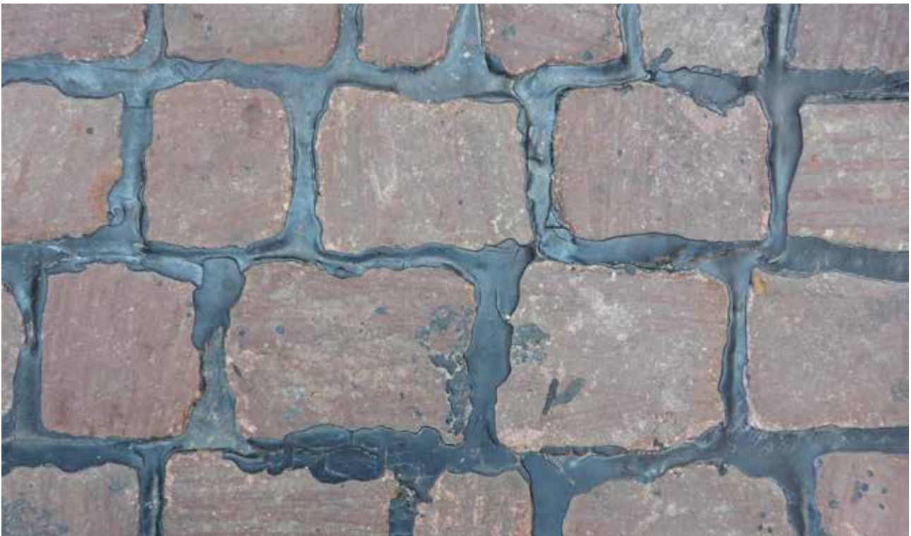
Bike friendly cobblestone treatment in Freiburg im Breisgau – similar measures could be applied in Ybbs an der Donau.
