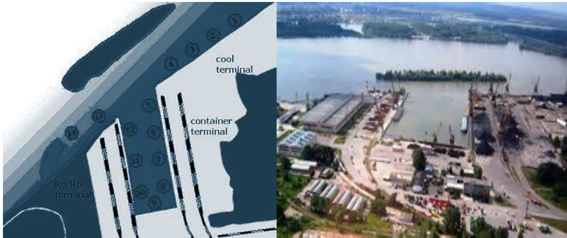
Figure № 5 Port terminal Ruse – East
