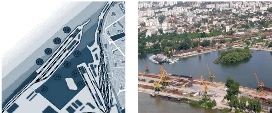
Figure № 6 Port terminal Ruse – West
