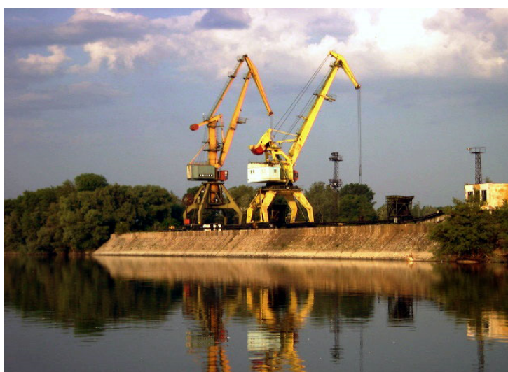
Figure № 16 Port terminal Vidin – South
