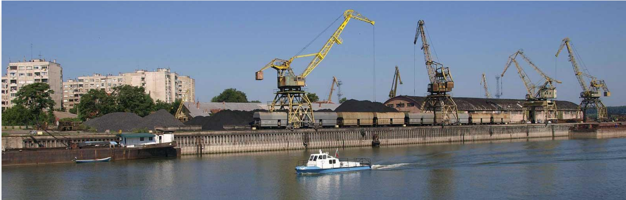
Figure 8: Port terminal Lom
