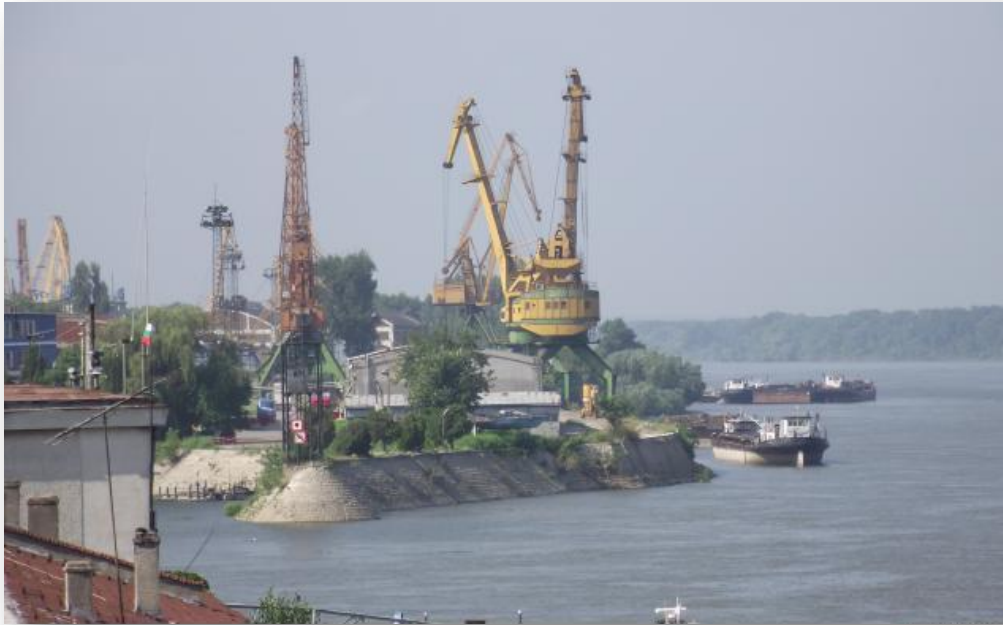
Figure 3: Port terminal Ruse-west
