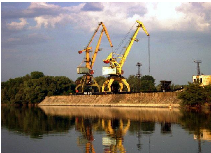
Figure 12: Port terminal Vidin – South
