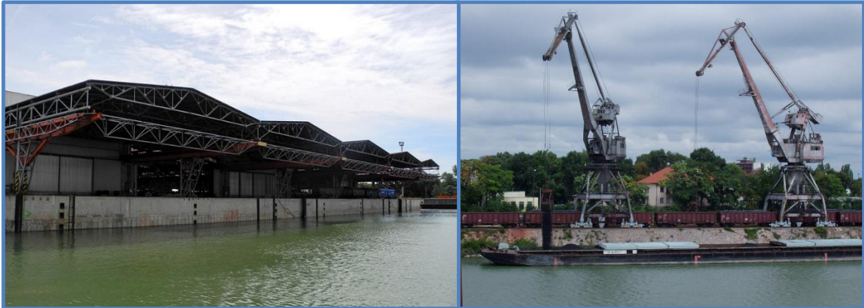
Figure 15: Port of Bratislava (left) and Komarno (right)
