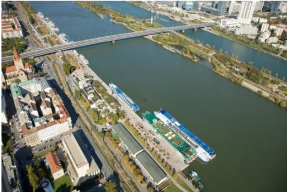
Figure 11: Port of Vienna – passenger terminal
