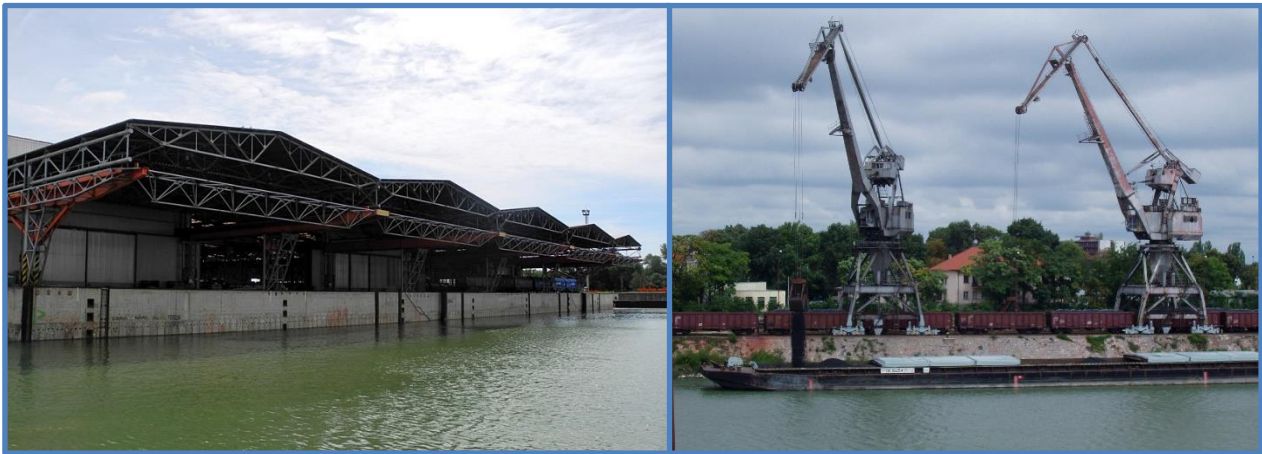
Fig. 8 Port of Bratislava (left) and Komarno (right)
