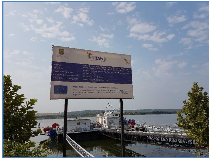
Figure 14: Residues receiving system in the Port of Drobeta Turnu-Severin
