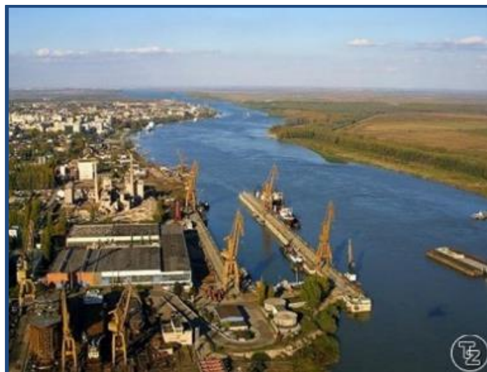
Figure 3: Port of Braila (Source: APDM)
