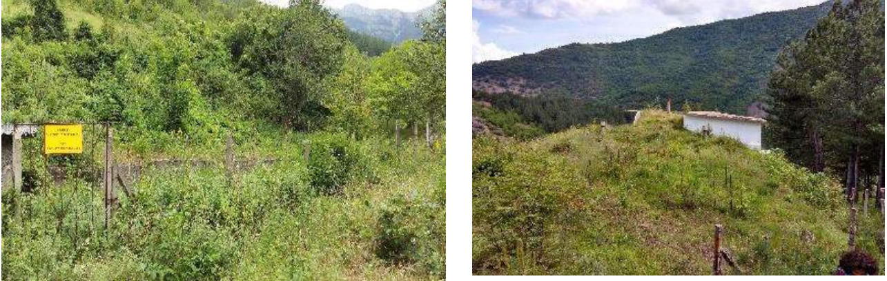
Fig. 2 Cross-sectoral cooperation between water and forest authorities in drinking water protection areas in Bulgaria, pilot area – watershed “Ochindolska reka”, © EFA
