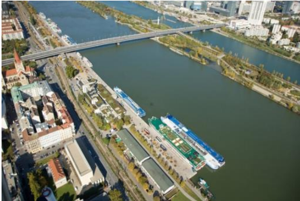
Figure 11: Port of Vienna – passenger terminal
