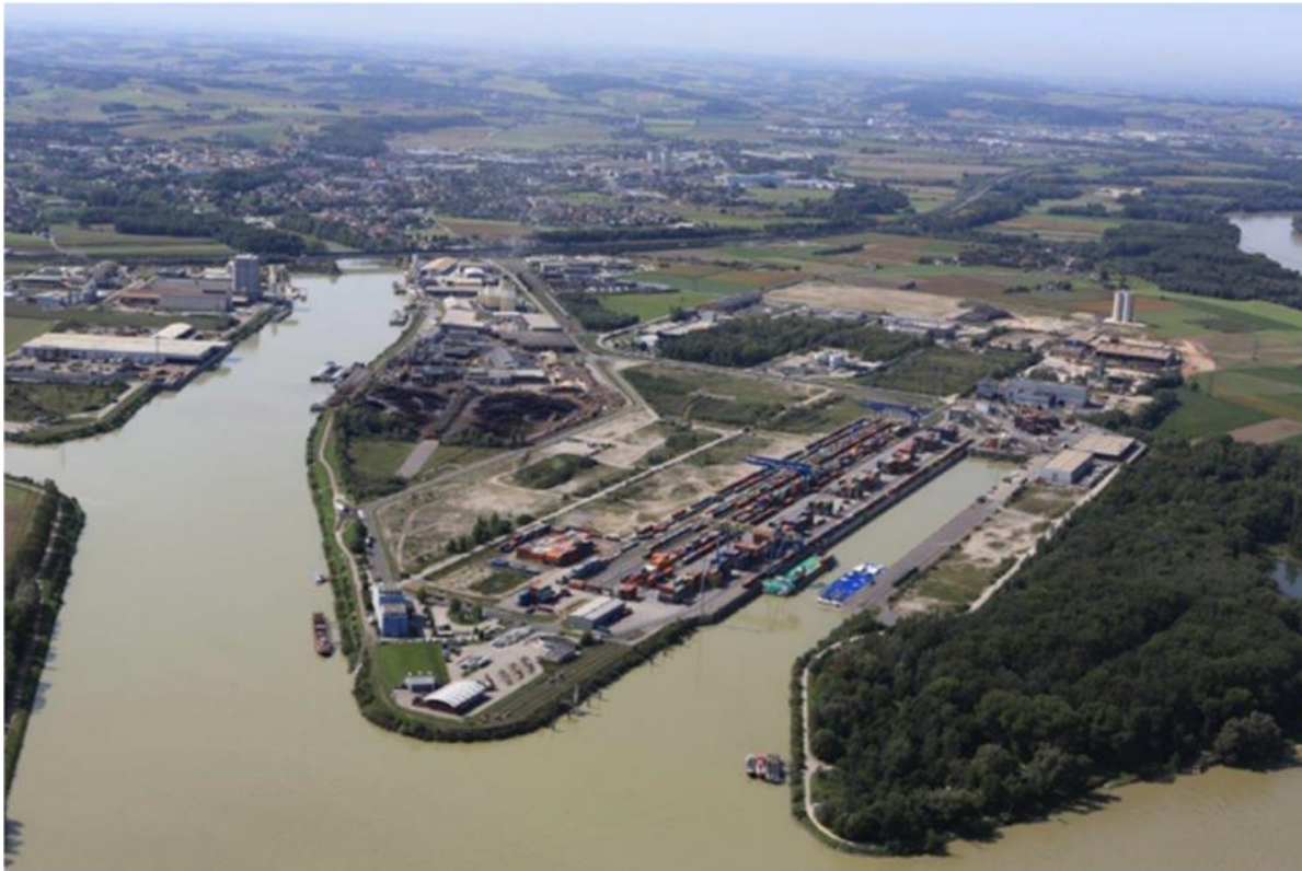
Figure 2: View of the Port of Enns
