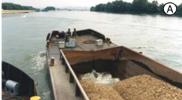
Granulometric River Bed Improvement. Approx. 120.000 m 3 of coarse gravel
