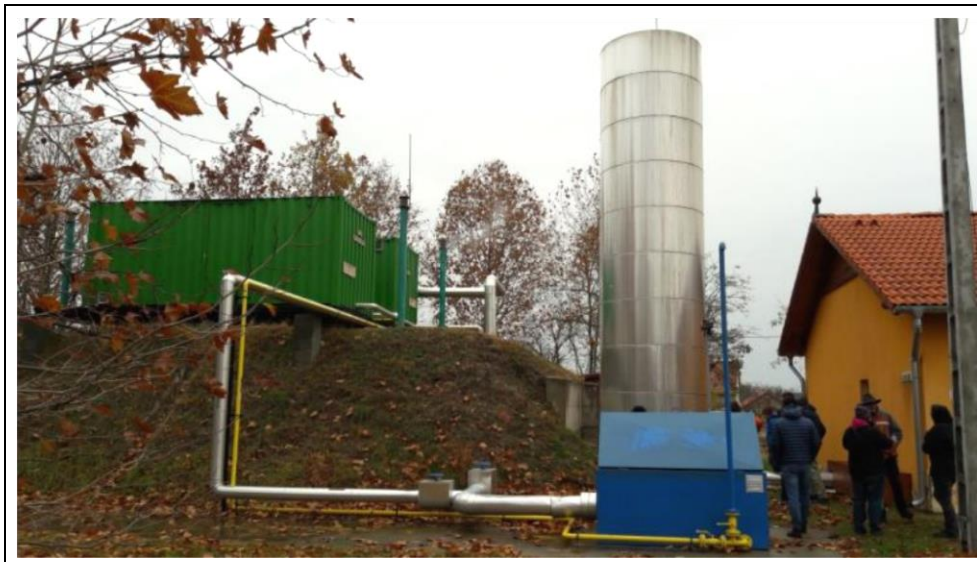
Figure 27: The production well (B-45) and the gas separator in the Hunyadi Park, Mórahalom, Hungary
