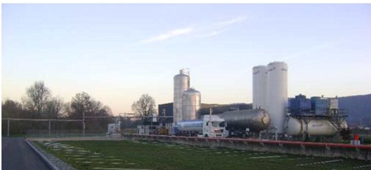
Figure 33: Messer BH gas d.o.o, Republic of Srpska, extraction of CO 2 from thermomineral waters
